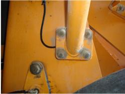
Light support bracket bolts after 2yrs- 1 recoat.
